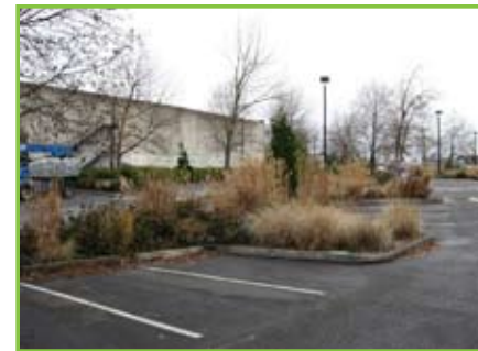
Curb cuts in the vegetated swales, along with the grade of the lot, encourage water to enter the swale. This is located at a parking lot for the Oregon Museum of Science and Industry.
