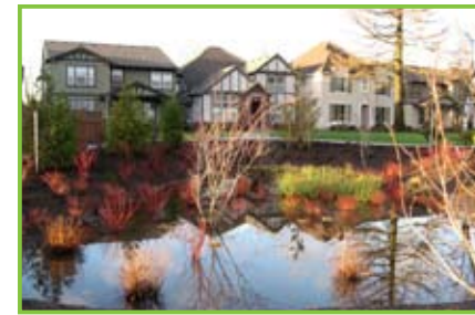
Villebois is a large neighborhood development in Wilsonville, Oregon, that incorporates decentralized stormwater management features throughout. Larger retention ponds were the solution to building codes that don't allow rain gardens close to home foundations.
