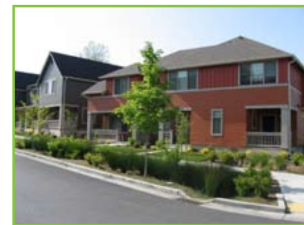
Curb cut and swale at High Point in West Seattle.
